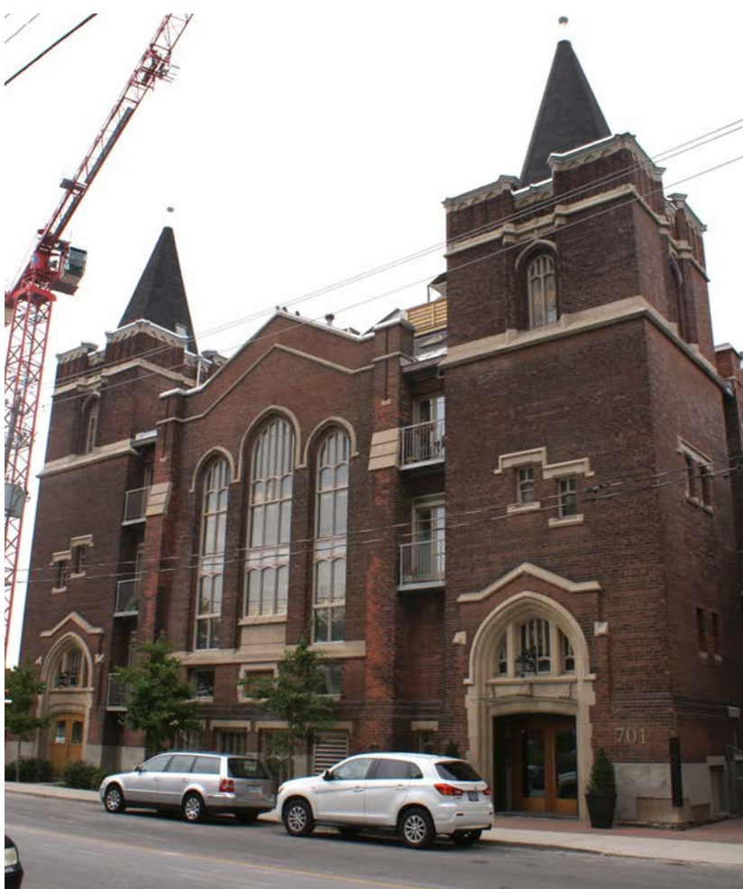
The Church Lofts 701 Dovercourt Road
