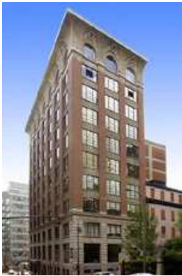
Fig.9 The 1912 Unity Building designed by David Jerome Spence for the
